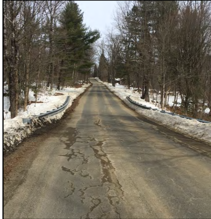
Road Above Culvert
